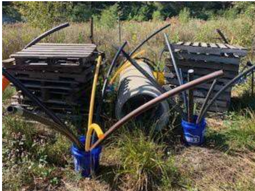
Figure 2 – Example of pallet tower, spider bucket and reinforced concrete culvert pipe.
