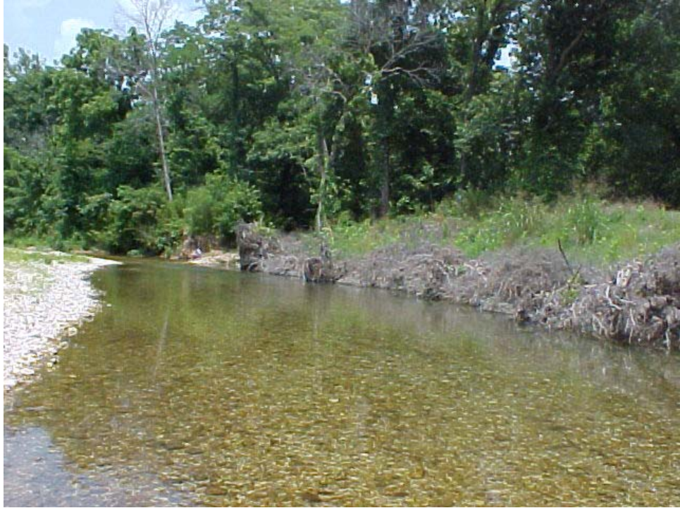
Figure 1. Picture of completed cedar tree revetment at Spring Creek in northeast Oklahoma.
