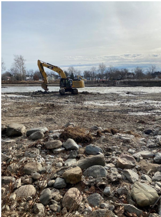
Pictured above: Post removal of Logansport Dam
