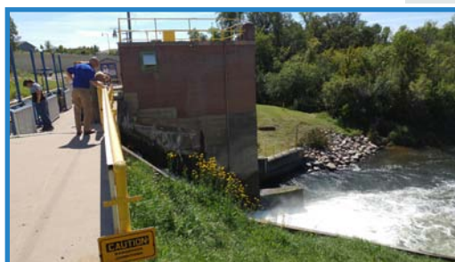
A tour of the 5 Otter Tail Power hydroelectric dams with OTP, FERC, and DNR. This is Pisgah Dam.
