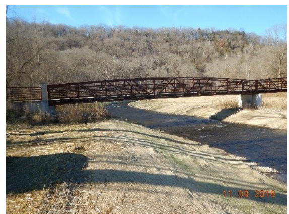
The completed channel realignment with sloped & seeded banks.
