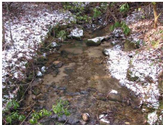
Brook trout stream in February 2007 during initial phase of residential subdivision road construction.
