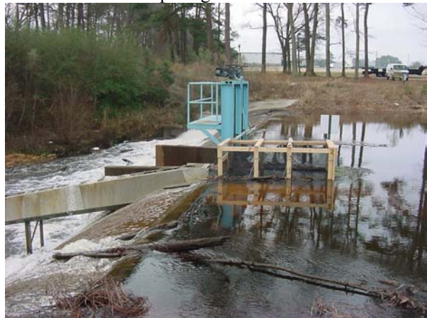
Holts Lake dam fishway.
