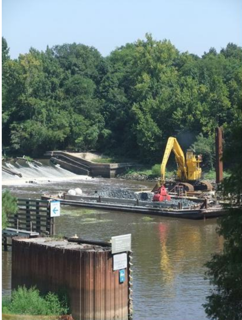
Scour hole filling below Cape Fear River Lock and Dam #1
