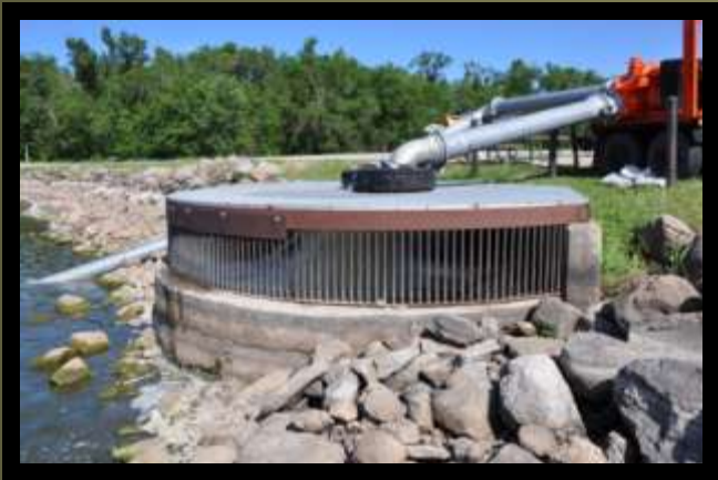
Godwin pump moving water off of Swan Lake.
