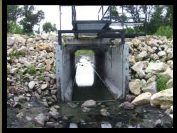
The old outlet structure at Lizard Lake (left). The new outlet structure at Lizard Lake with all of the stop logs removed to allow the lake to drain (right). The elevation of the new structure (with all stop logs in place) matches the elevation of the old outlet at the bottom of the notch.
