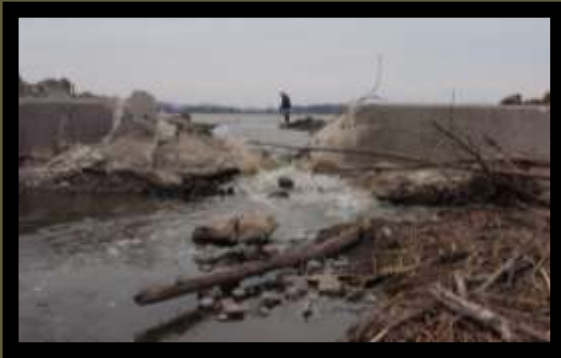
April 2011. Draining of Pickeral Lake and removal of old outlet structure.
