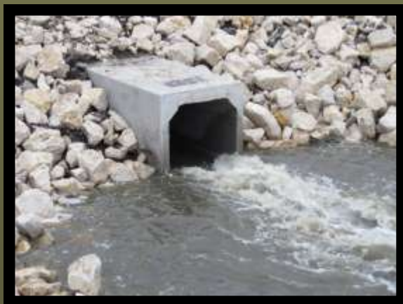
The old outlet structure at Lizard Lake (left). The new outlet structure at Lizard Lake with all of the stop logs removed to allow the lake to drain (right). The elevation of the new structure (with all stop logs in place) matches the elevation of the old outlet at the bottom of the notch.
