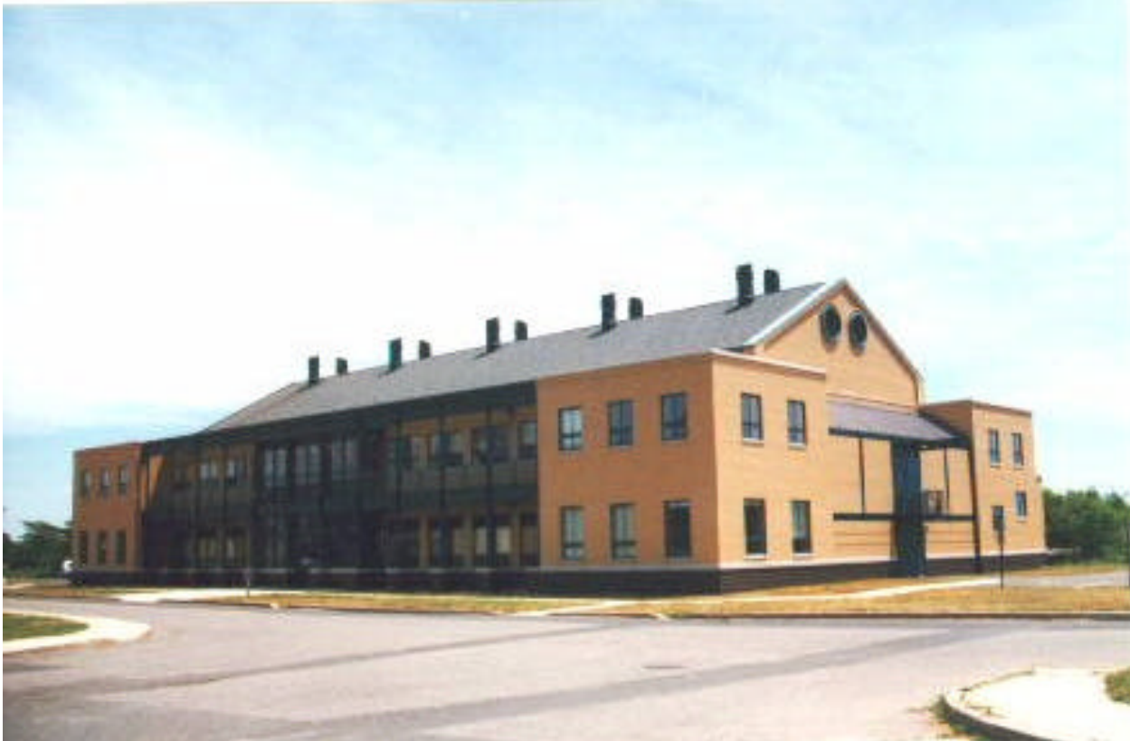
The new NMFS laboratory at Sandy Hook, NJ. The new 32,000 sq ft laboratory housing experimental seawater, analytical chemistry, and microbiology laboratories is directly across the street from the renovated 35,000 sq ft converted Army barracks that houses offices, conference rooms, and the Lionel A. Walford Marine Science Library. The new laboratory was completed in October 1993. Renovation of the historic 1890s army building was completed in 1994. Design of the new building and renovation of the old were carefully planned to retain the unique historical character of Fort Hancock (a historic landmark), while meeting rigorous technical standards demanded by scientists and conforming to environmental and safety requirements.
