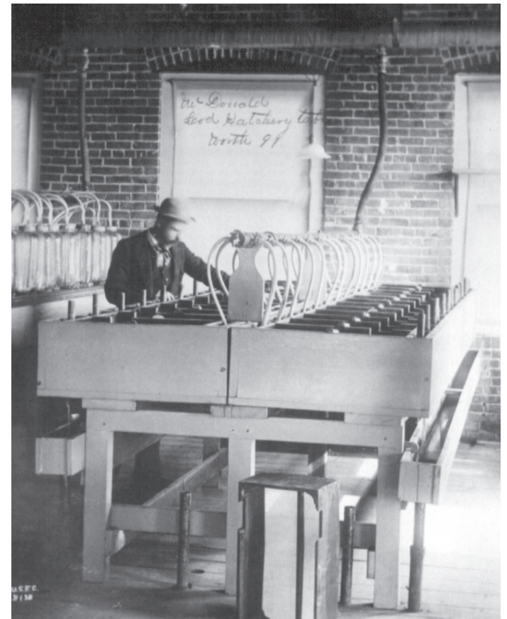
Cod hatching table at U.S. Fish Commission hatchery at Woods Hole Station. McDonald hatching tests. Marshall McDonald was president of AFS 1885–1886. Worth photo 1891. NOAA NORTHEAST FISHERIES SCIENCE CENTER
