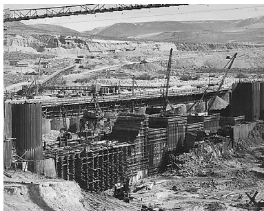
Construction of Grand Coulee Dam, Columbia River Basin, 1936. NATIONAL ARCHIVES
